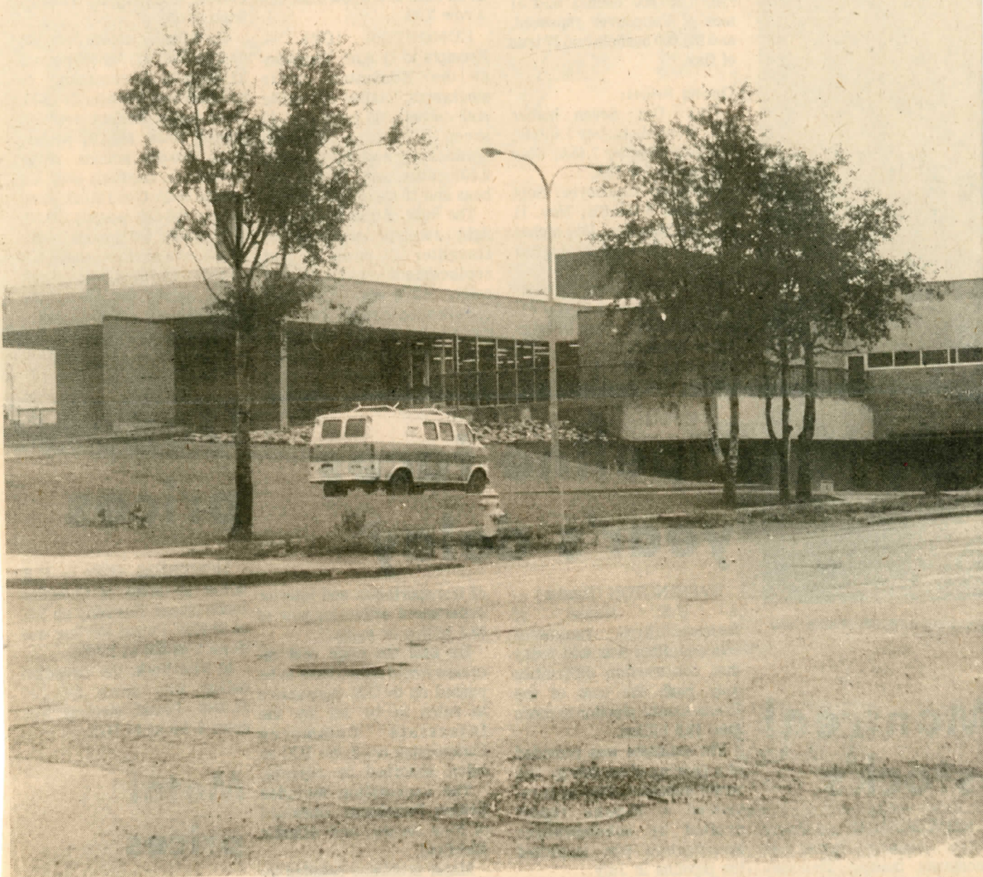
THE NEW EXTENSION to the Fort St John General Hospital was completed substantially on June 15. Since then it has been landscaped and the interior
