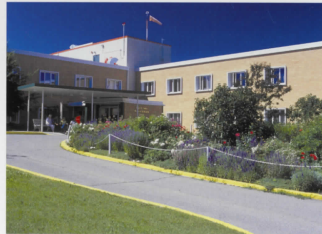
FORT ST. JOHN HOSPITAL
