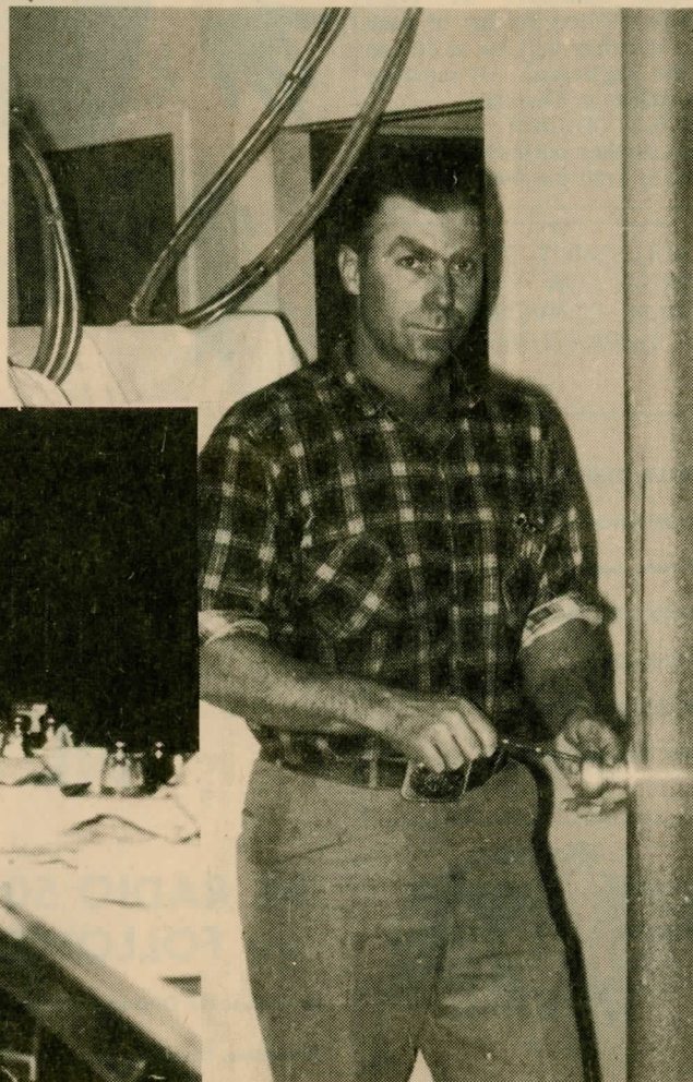
RAY SOWDEN, CARPENTER, is busy putting the finishing touches to the new X Ray room in the hospital. Completely new X Ray equipment has recently been aquired.
