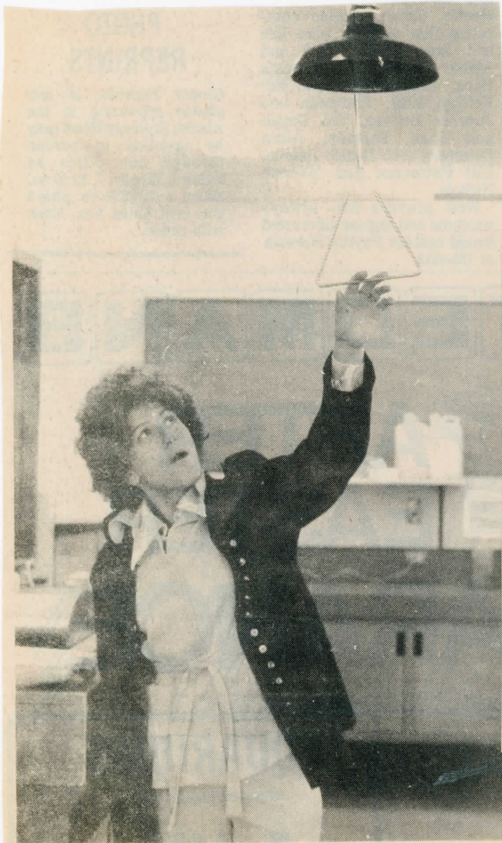
LAB WORKERS SPRAYED with dangerous fluids can use this emergency sprinkler in the new laboratory. Hospital Trustee Regina Schaerer said that safety had been a prime consideration in its design.
